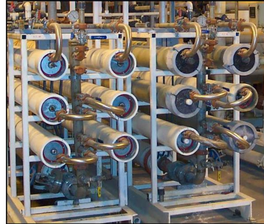
Reverse Osmosis Units
